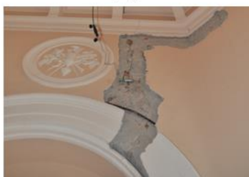
Figure 2.11. a) Damage survey of the Osservatorio Vesuviano Tower; b) damage detail on vaulted
