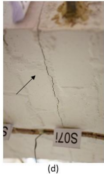
Figure 6.16. Arch damage: a) view of crack location; (b) crack C1; c) crack C2; d) crack C3
