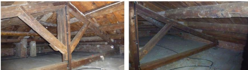
Figure 5.11. View of the wooden trusses
