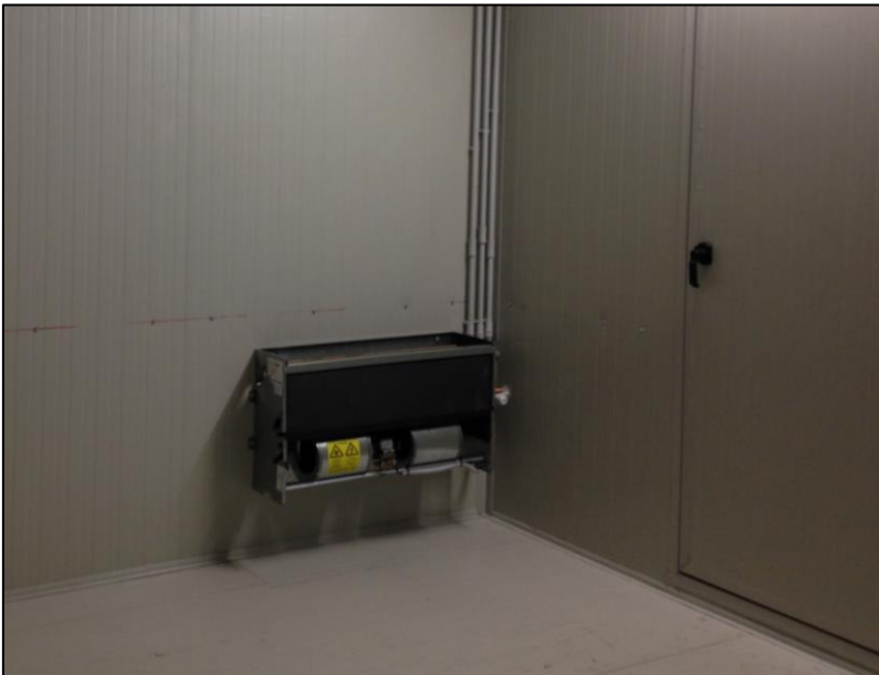
Figure 6: fan-coil reproducing summer temperature values.
