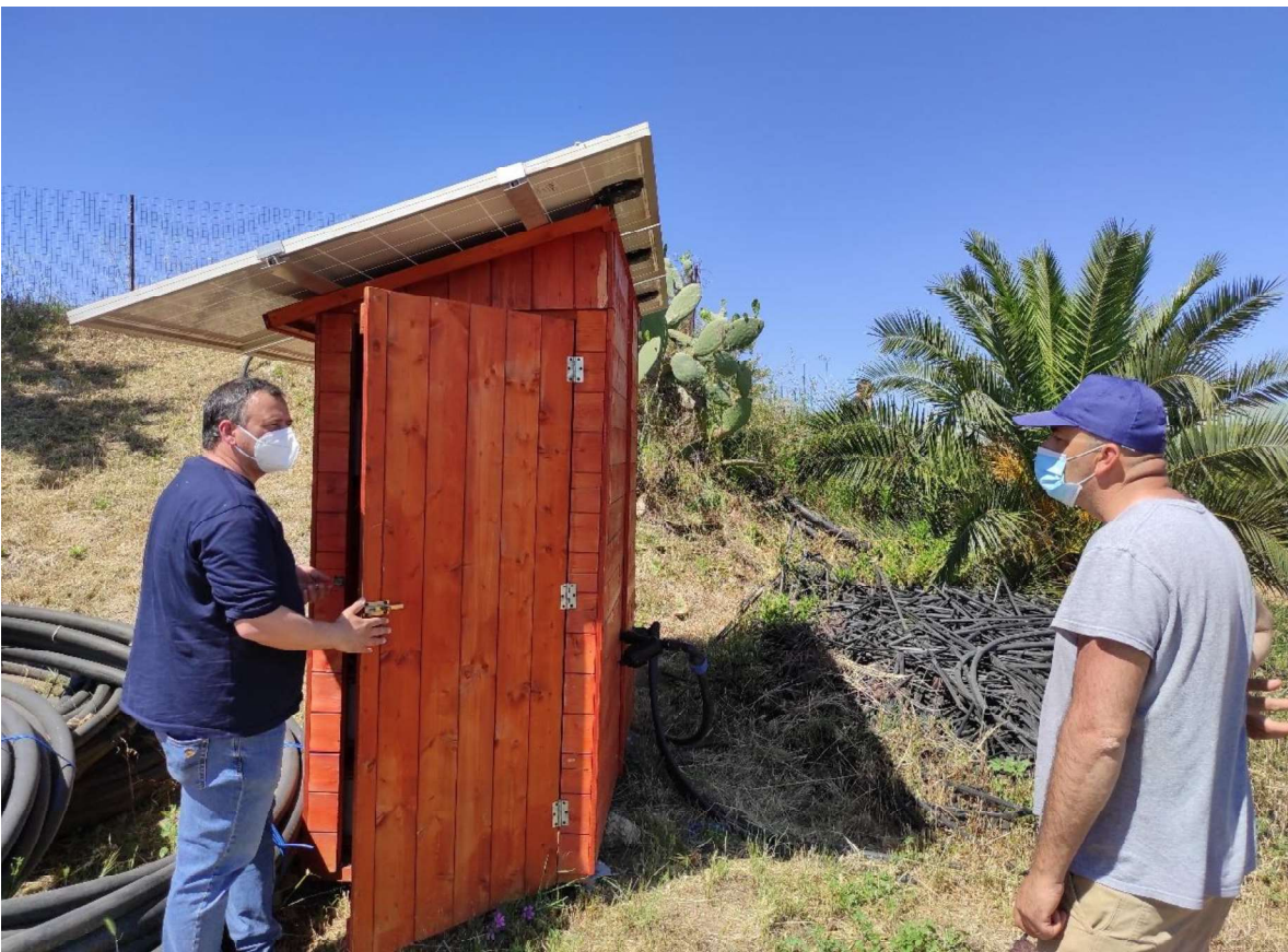
Figure 3.41. Solar fertigation system installation at region-3 (Apulia region).
