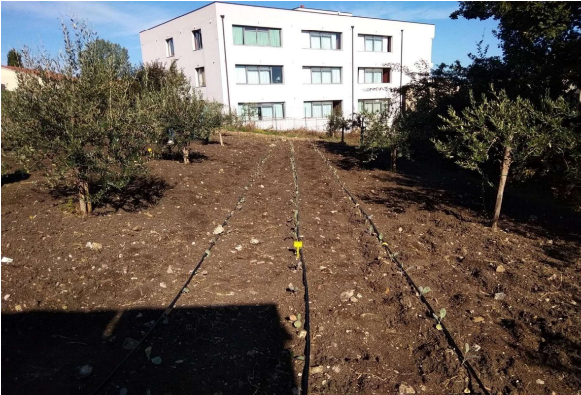
Figure 3.26. Solar fertigation system installation at region-1 (Molise region – Campobasso).
