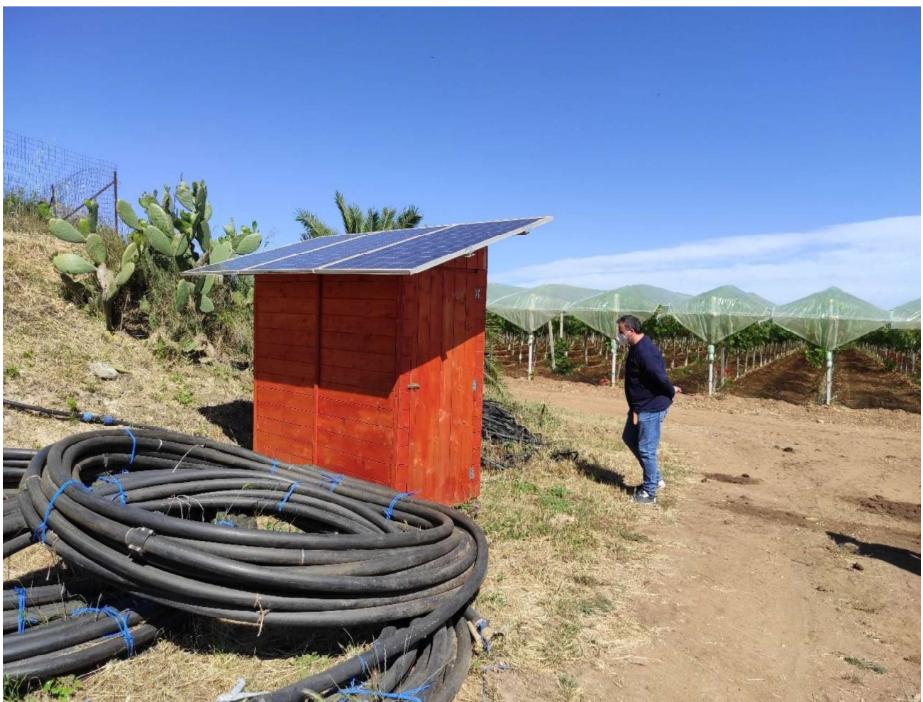
Figure 3.39. Solar fertigation system installation at region-2 (Apulia region).
