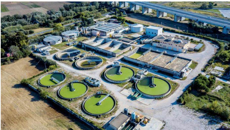
Figure 6.1 - Aerial view of the COSIB wastewater treatment.
