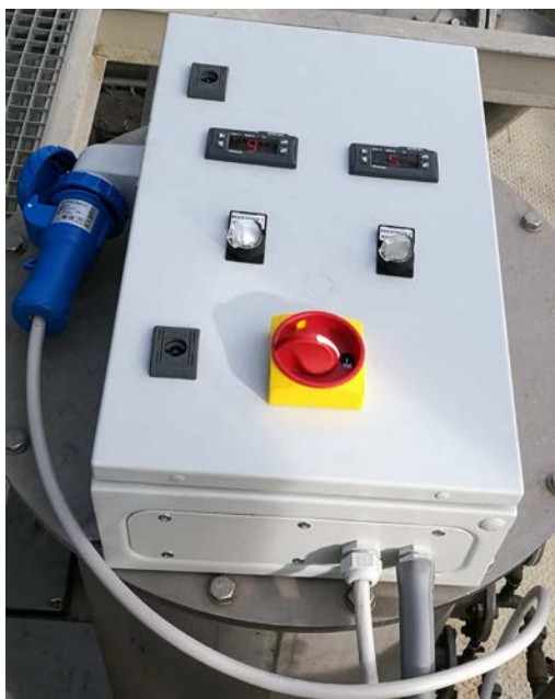
Figure 6.41 - Sampling probe drive panel.
